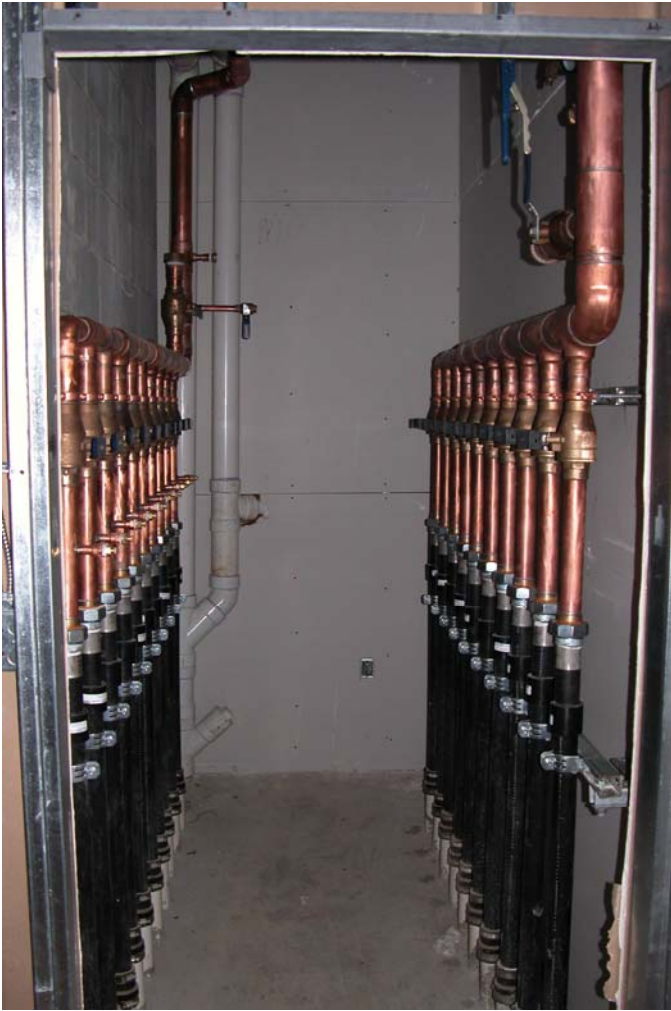
During Installation - Mechanical Room/Heat Pump
