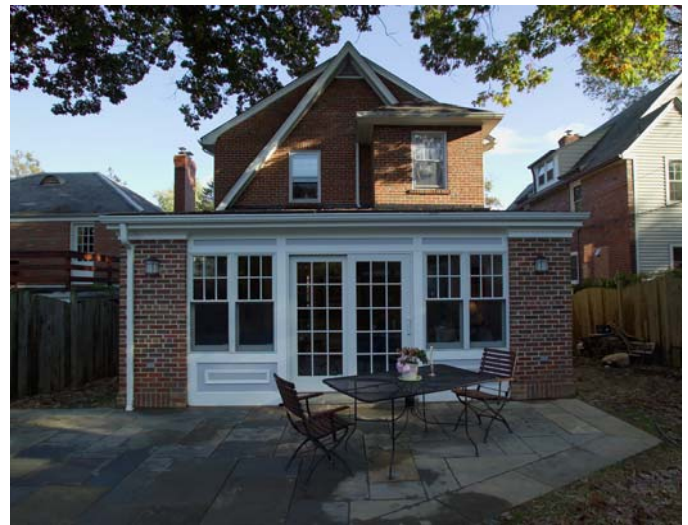
AFTER - VIEW OF REAR FAÇADE & STONE PATIO
