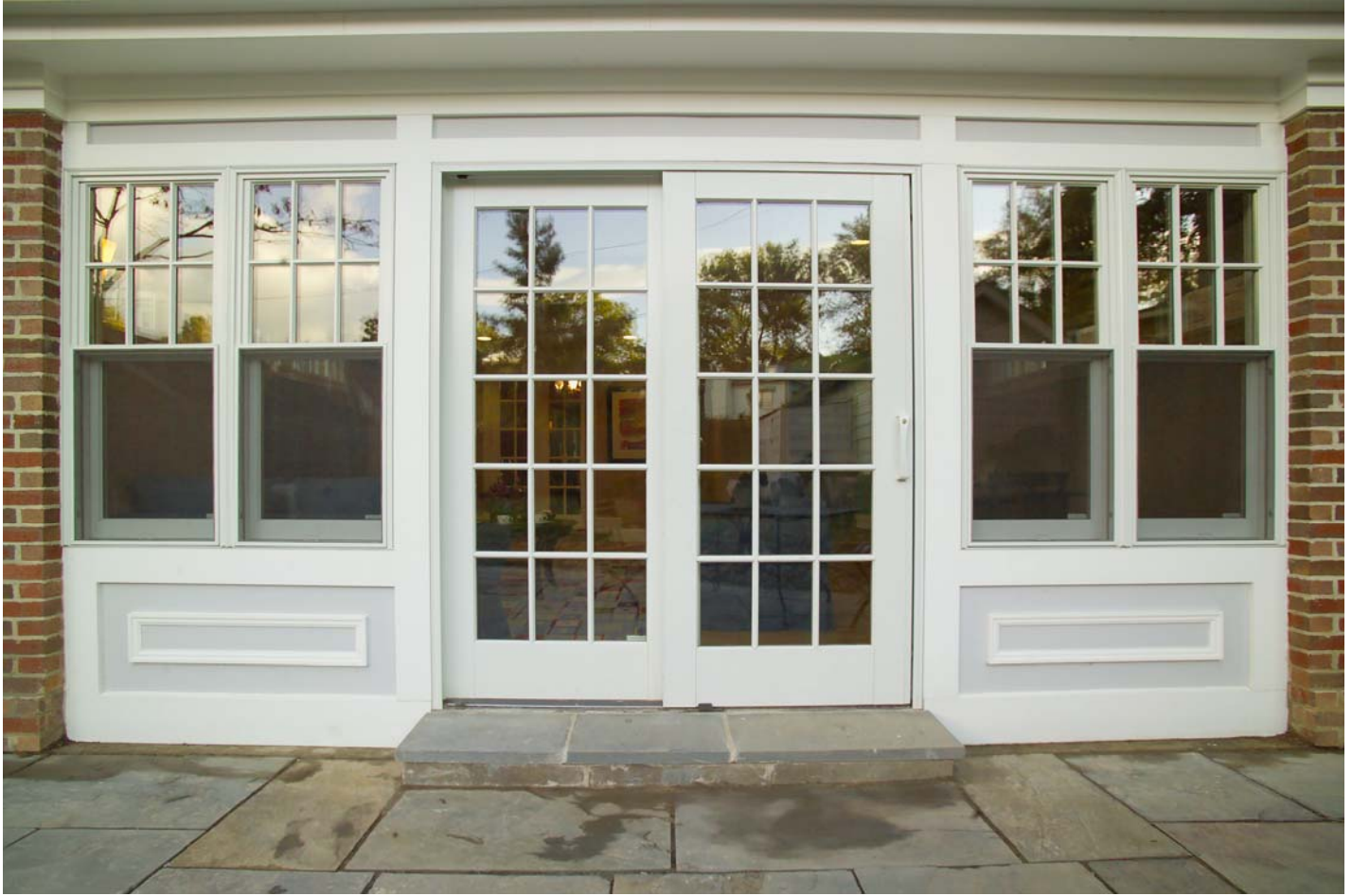
AFTER - VIEW OF REAR FAÇADE & STONE PATIO “The exterior of the addition uses both brick and Hardi panel siding. Inset panel molding accents the fenestrations”
