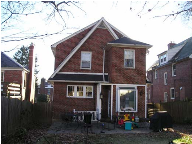
BEFORE - VIEW OF REAR FAÇADE
