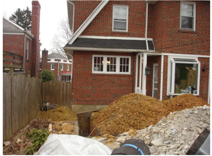
DURING - VIEW OF REAR FAÇADE – Prep for new foundations
