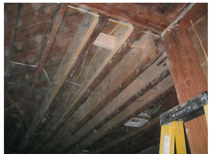
DURING PICTURE – Sister joists below Master bathroom.
