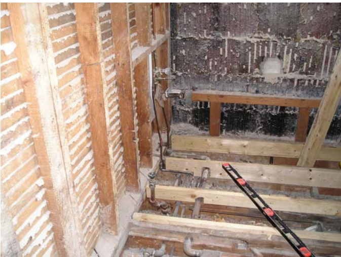
BEFORE PICTURE – Existing conditions of Master bathroom previous to start work.
