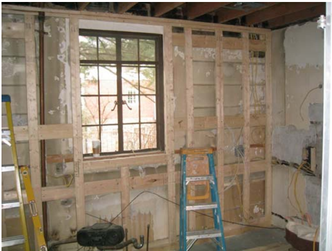
DURING PICTURE – View Of Casement Window Above Sink During Construction.
