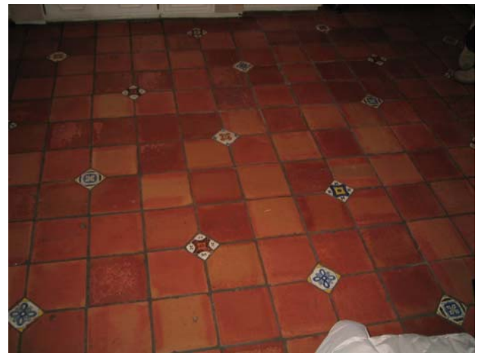
BEFORE PICTURE – View Of Existing Floor Tiling.
