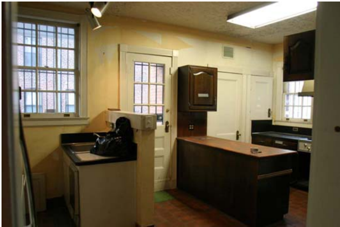
BEFORE PICTURE – View of existing peninsula, sink & kitchen's back door.
