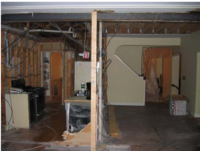
BEFORE PICTURE – Existing kitchen conditions after demolition by previous contractor.
