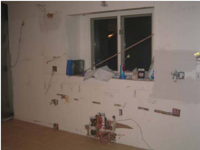
DURING PICTURE – View Of Window Above Sink.
