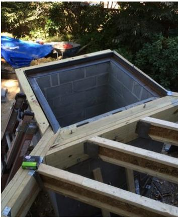
Concrete block framing for the base of the pizza oven.
