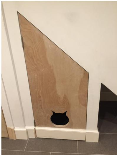
Lead carpenter Carlos Marin was working on an under stair closet for the litter box for two cats when the client asked him to make a cat-shaped opening. He created a template using a flower pot to trace the circle and wood triangles for the ears. A quick cut with a jigsaw and the cat door was ready. The closet is in a basement laundry area. We also installed a motion detector vent fan in the room.
