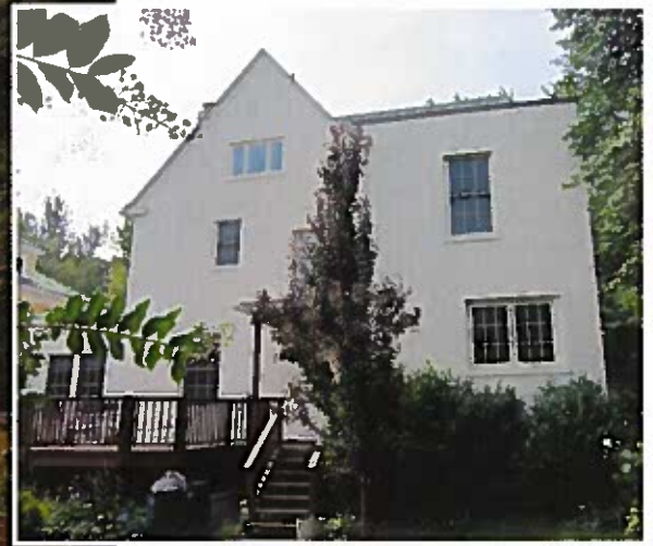
The original home is stucco (inset), which has a heavy look. Landis matched the stucco and used it on the addition, but to lighten the feel and add interest, the company used fiber cement HardiePanel and trimmed it with a composite product called Tru Exterior (left). The differing shades of paint on the HardiePanel and the trim add depth to the exterior.
