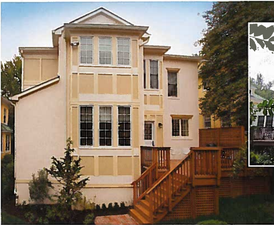
The original home is stucco (inset), which has a heavy look. Landis matched the stucco and used it on the addition, but to lighten the feel and add interest, the company used fiber cement HardiePanel and trimmed it with a composite product called Tru Exterior (left). The differing shades of paint on the HardiePanel and the trim add depth to the exterior.
