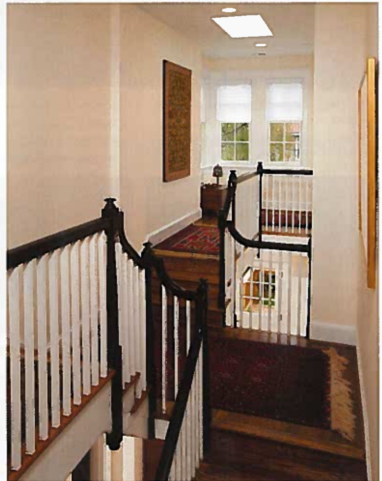
The windows in the landing face the north, so adding a skylight brings in more natural light. A millwork subcontractor copied the design of the original stair railing and posts for the new landing.
