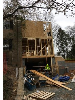
IN PROGRESS: 1st and 2nd floor framing over the widened garage.
